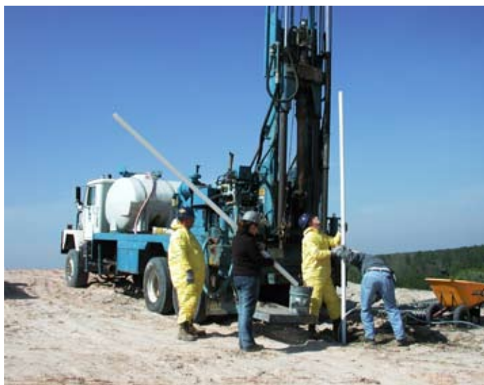
Vertical wells were drilled at the New River bioreactor. Small diameter pipes (PVC; 2 inches in diameter) were placed into holes constructed with an open-flight rotary auger (4.5 inches in diameter).
